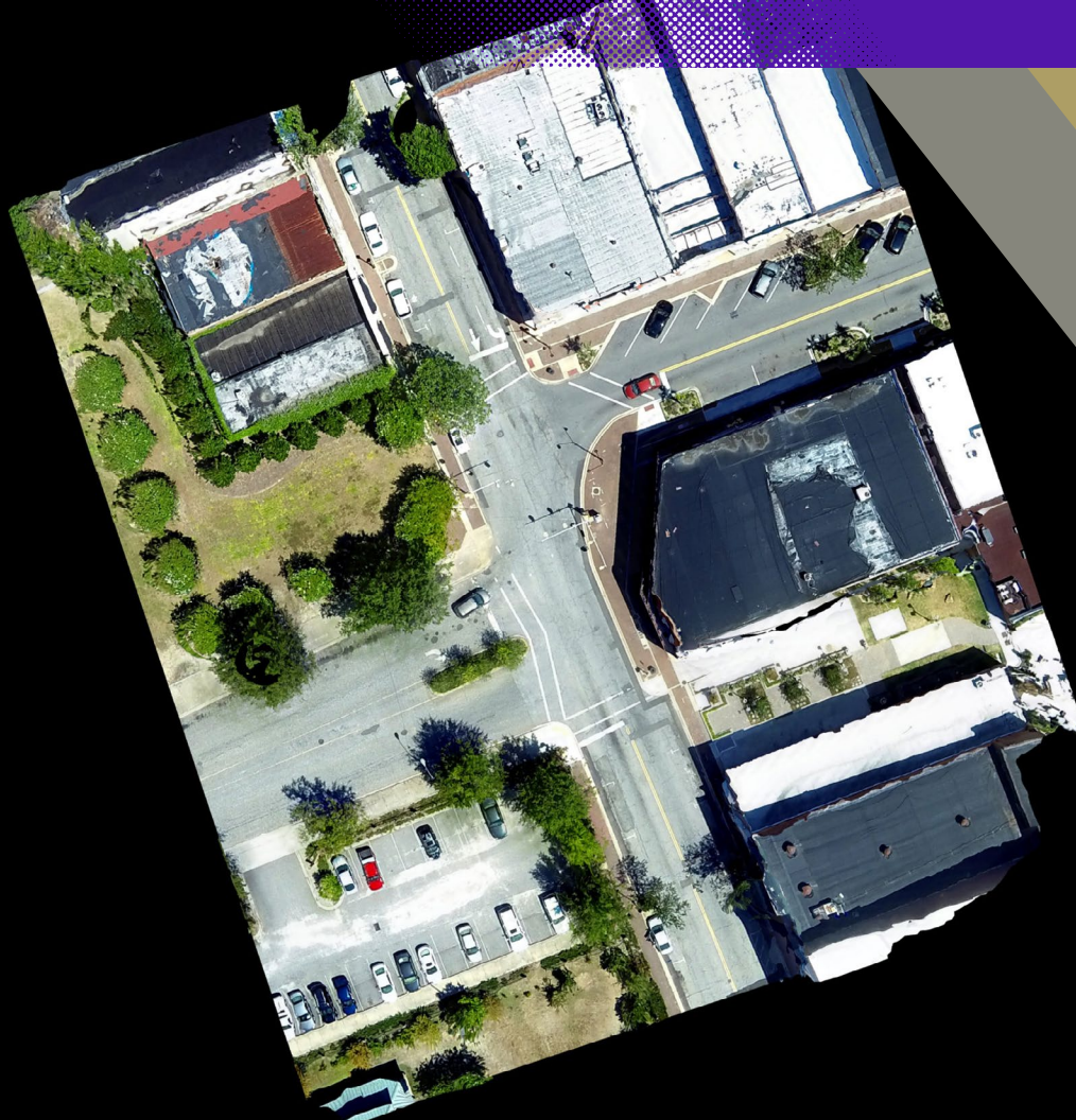
True orthoimage created with a drone.
