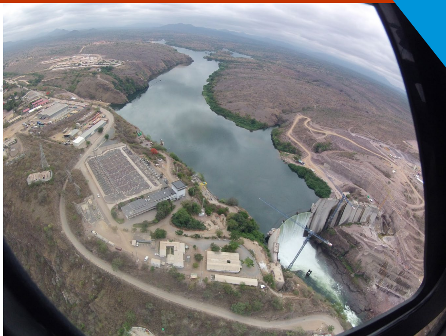
Main operating base at Hydro Electric plant
