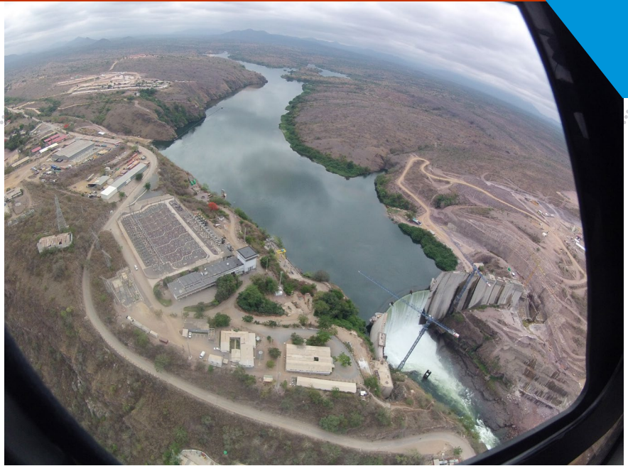
Main operating base at Hydro Electric plant
