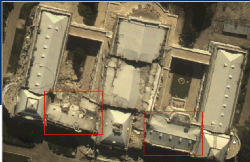
Figure 1A High spatial resolution imagery, showing the damage to the Presidential Palace.
