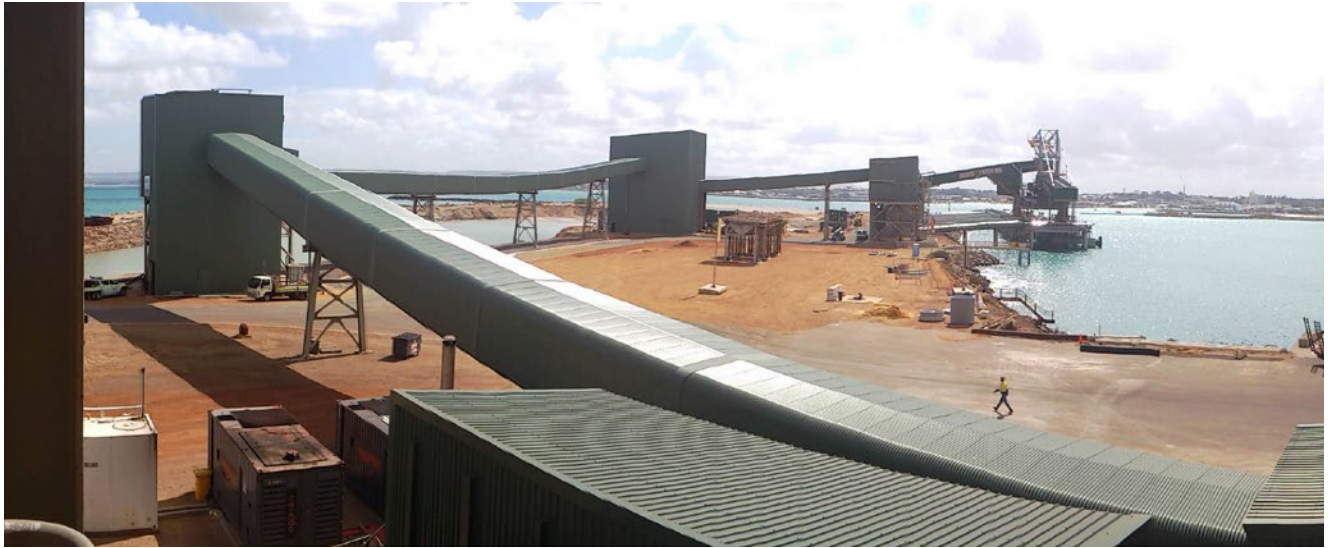
From the Karara holding shed iron ore is transported directly to ships via a side conveyor.
