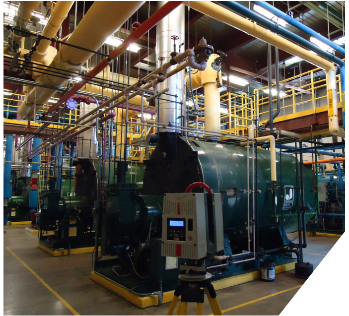
Upstate New York Boiler Room Modification Project
