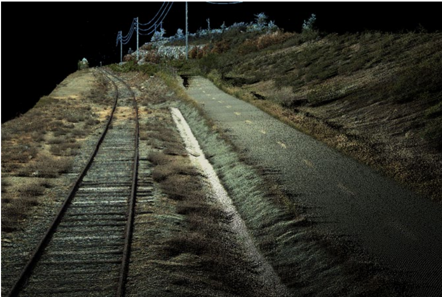
Sacramento Valley Rail line Mobile LiDAR survey from Historic Folsom.
