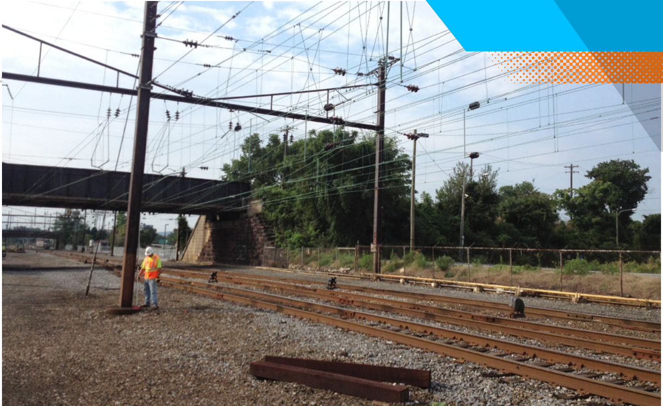
An SSI field surveyor occupying a control point in establishing the project control network. SSI set pairs of EMATs (Elevated Mobile Acquisition Targets) at 300 foot intervals over the entire project area.
