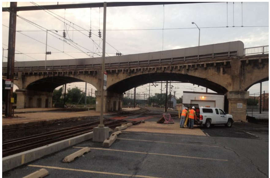
SSI survey field crew establishing the mobile mapping control network on the project area. The coordinate values were utilized to control the LiDAR dataset to maintain engineering design tolerances.
