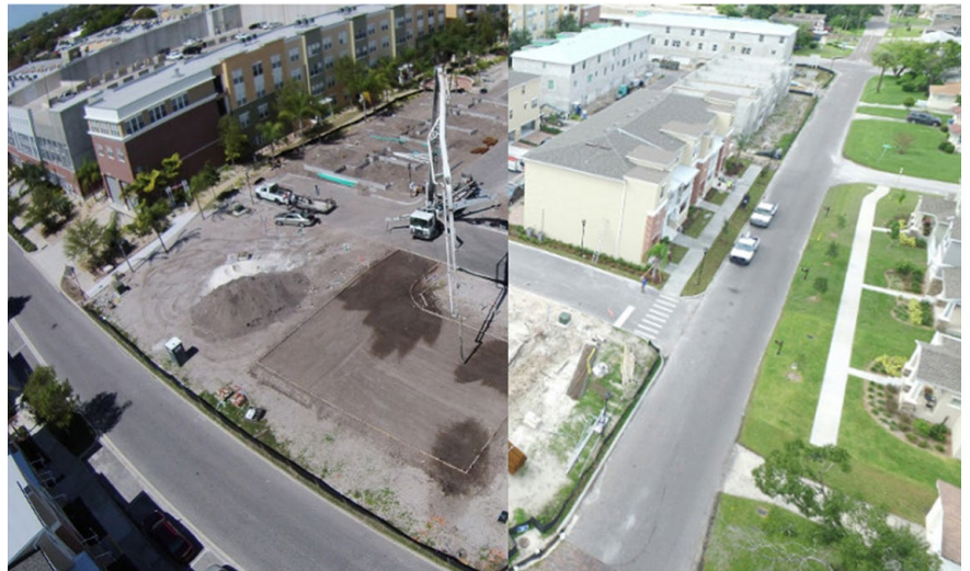
Below: Construction site monitoring is a very popular use for UAS. The image on the left was captured in February with a Phantom 2. The image on the right was captured with a Phantom 3 in September. Note the fisheye look in the Phantom 2's image on the left.
