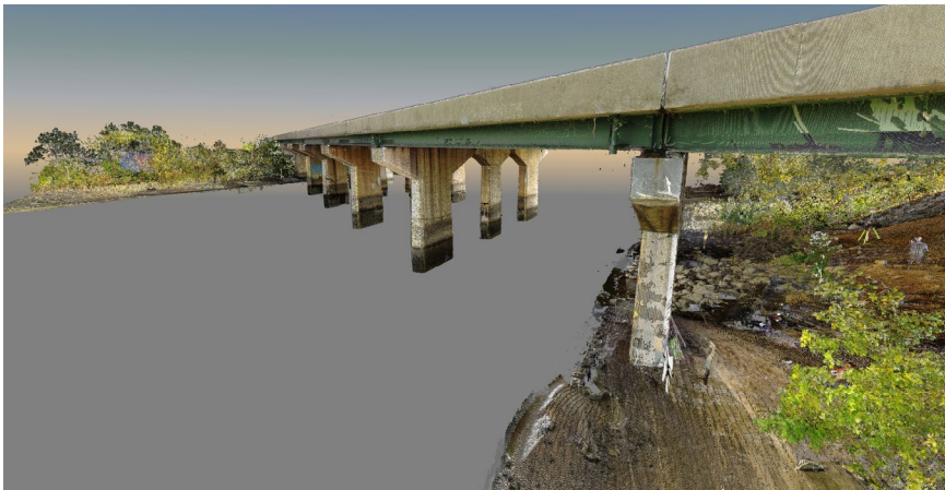
View of the bridge in Bentley Pointools
