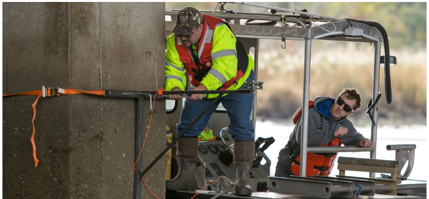
Installing the Jig on a pier
