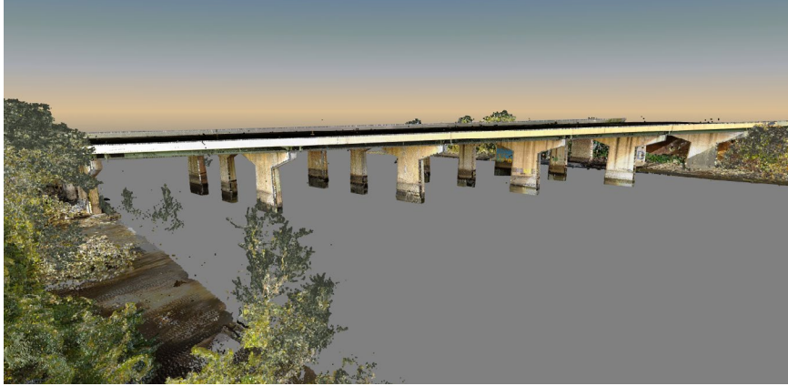
View of the bridge in Bentley Pointools
