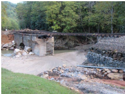
Damaged bridges, washed-out approaches and unstable terrain were among the conditions McKim & Creed survey teams encountered while documenting five NCDOT bridge sites in Buncombe County following Hurricane Helene.
