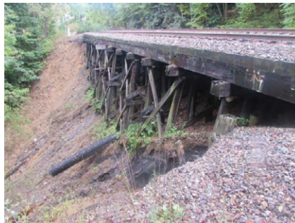
Damaged bridges, washed-out approaches and unstable terrain were among the conditions McKim & Creed survey teams encountered while documenting five NCDOT bridge sites in Buncombe County following Hurricane Helene.
