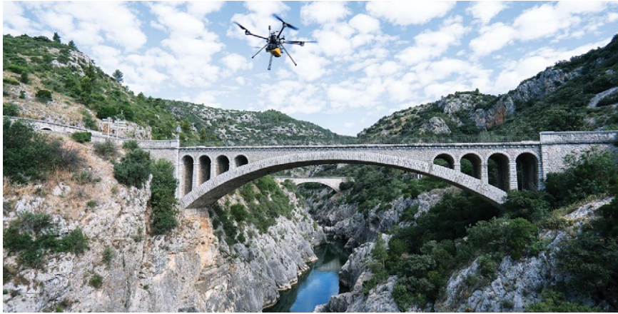
YellowScan Navigator topobathymetric lidar sensor deployed on a UAV above Le Pont du Diable, a bridge on the Herault river in France.
