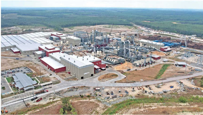
RoyOMartin's Corrigan manufacturing facility in Oakdale, Louisiana produces a variety of oriented strand board (OSB) panels.
