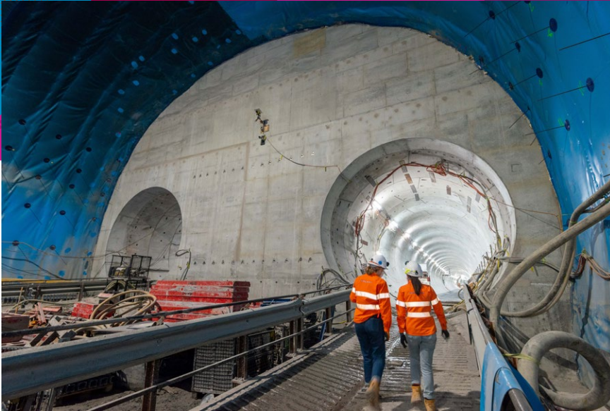
Workers enter the Roma Street cavern to conduct an inspection.
