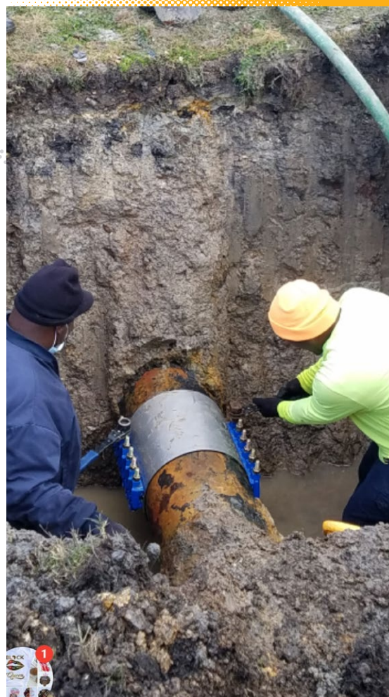
Images of an underground leak that was identified by ASTERRA in Greenville, Mississippi, after it was unearthed (left), and the subsequent repair (right).
