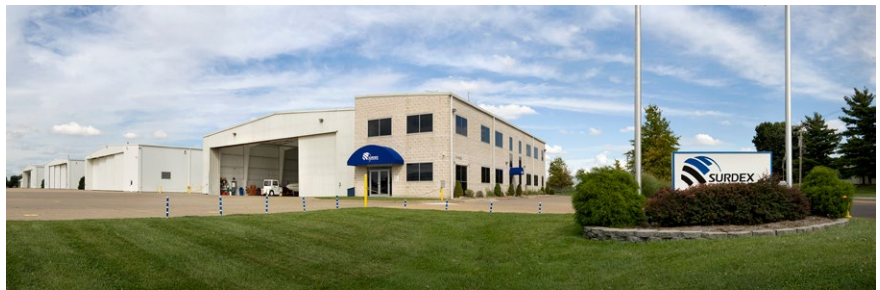
Surdex headquarters and hangar, Chesterfield, Missouri
