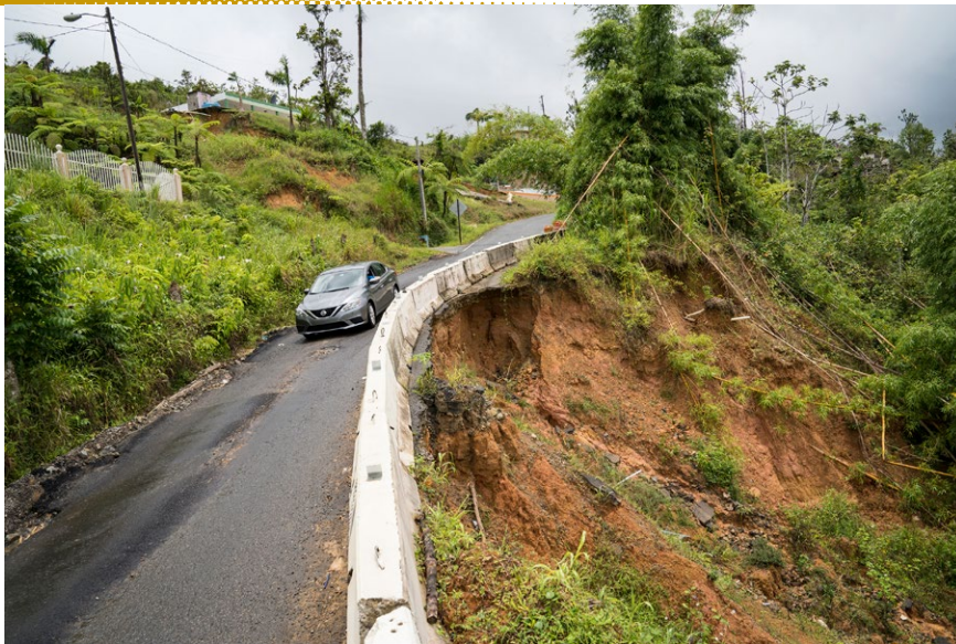
Many hillside roads in Puerto Rico were eroded by landslides after Hurricane Maria. Lidar data is being used to measure these elevation drops precisely and plan repairs.
