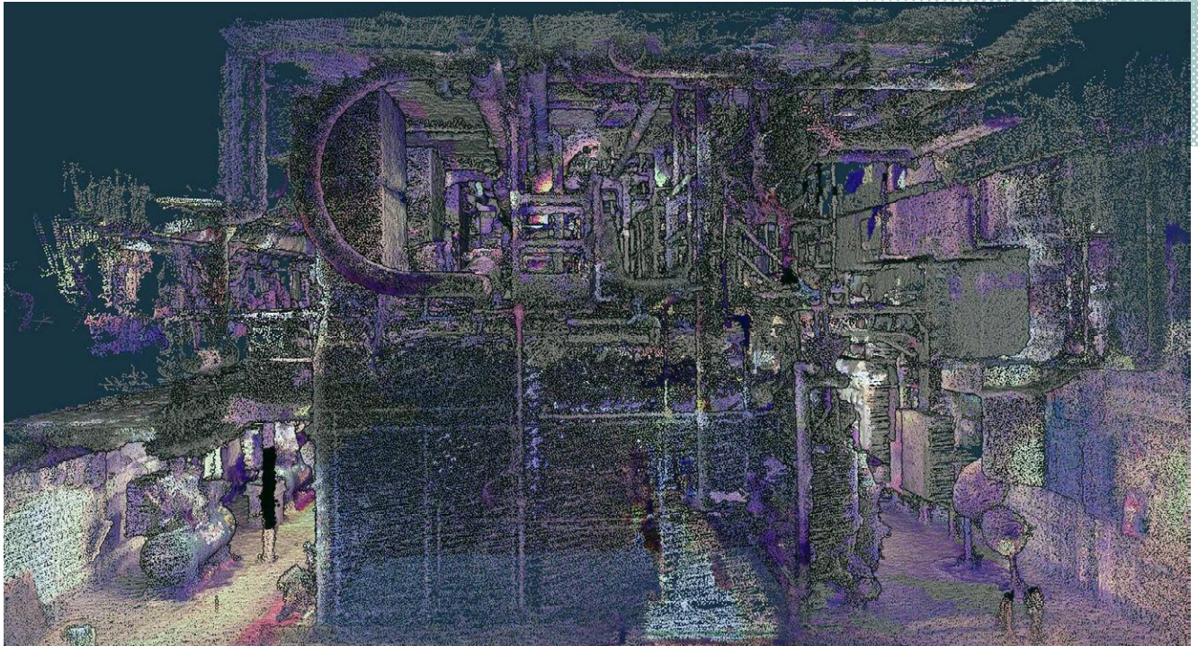
Figure 10: Colorized point cloud of tight spaces within hospital boiler room captured and processed with Kaarta Contour.
